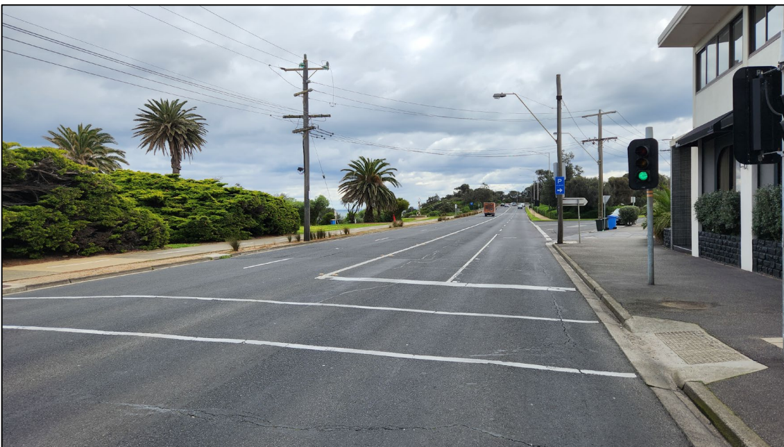
Figure 8 View of Beach Road facing north
