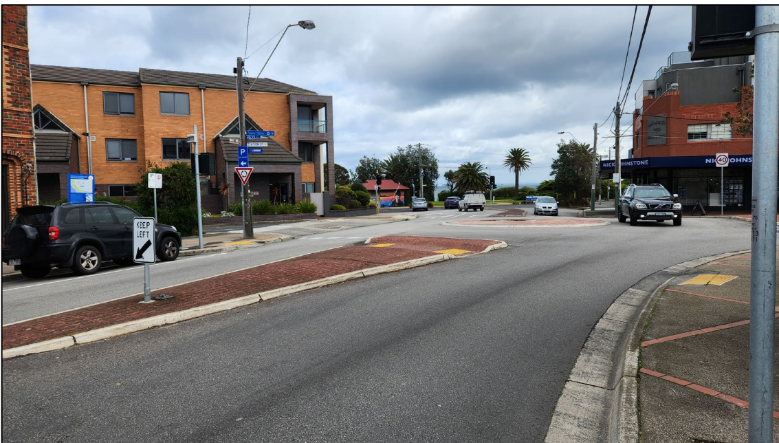
Figure 6 View of Bay Road facing west
