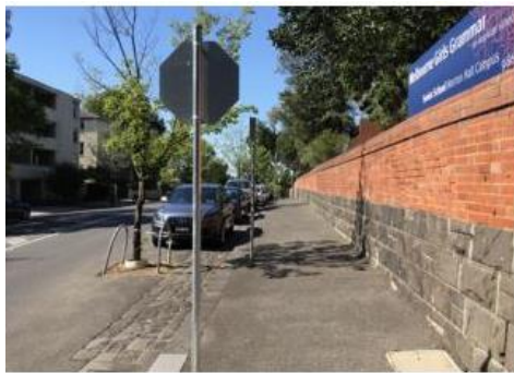
Original condition as a bitumen footpath (April 2017).
