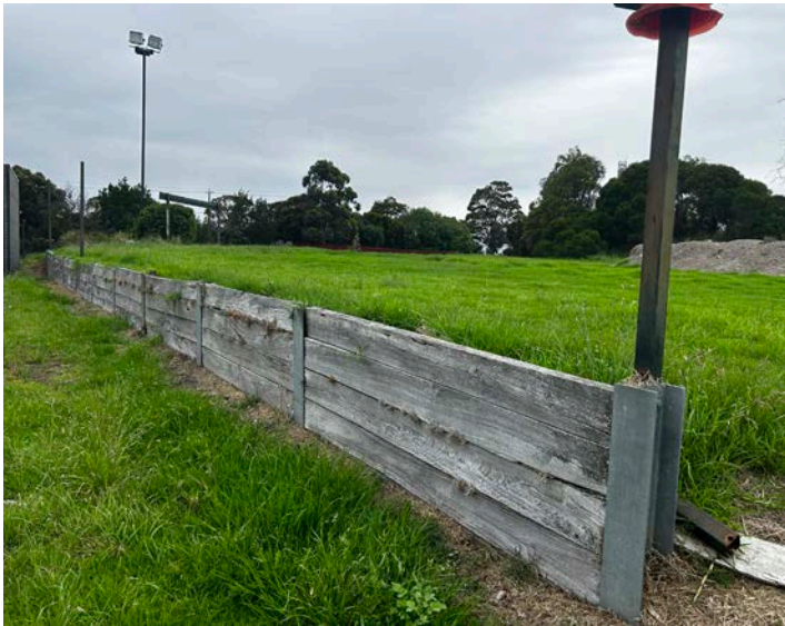
3 Timber retaining wall
