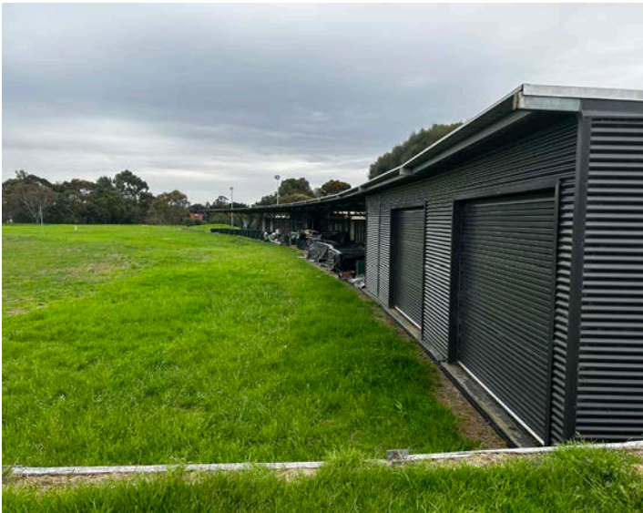
2 Existing infrastructure for previous driving range
