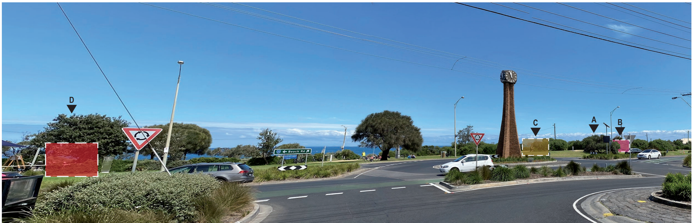
View 2 – Balcombe Road (east approach)
